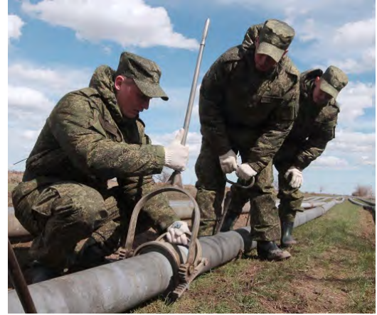
MTO Soldiers Laying Pipe
