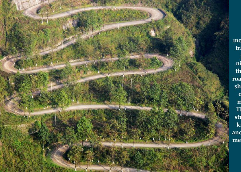
This mountainous track in the photo is nicknamed the "24-zig" road for its 24 sharp bends on a high mountain. The 24 zigs stretches 3.7 kilometers and has a 300meter vertical drop.
